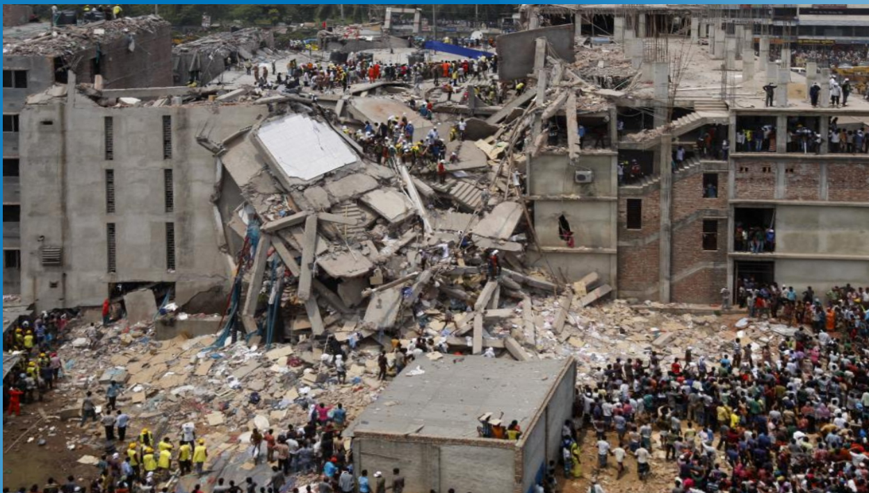
Wednesday, 24 April 2013, an eight-story commercial building named Rana Plaza, collapsed in Savar Upazila of Dhaka, Bangladesh. The search for the dead ended on 13 May 2013 with a death toll of 1,129. This image, originally posted to Flickr, was uploaded to Commons on 12 May 2013, by Rijans007. On that date, it was confirmed to be licensed under the terms of Creative Commons Attribution-Share Alike 2.0 Generic.
