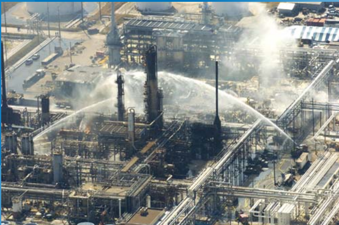
Fire-extinguishing operations after the Texas City refinery explosion. Attribute: Chemical Safety and Hazards investigation Board
